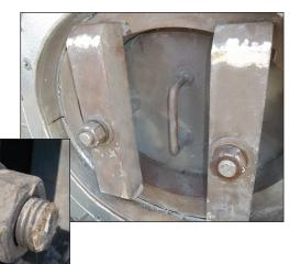
Chesterton's live loading technology includes an in-plant survey of steam drums and a complete engineering review of application parameters to select the proper gasket and improve gasket sealing stress through temperature and pressure cycling.
